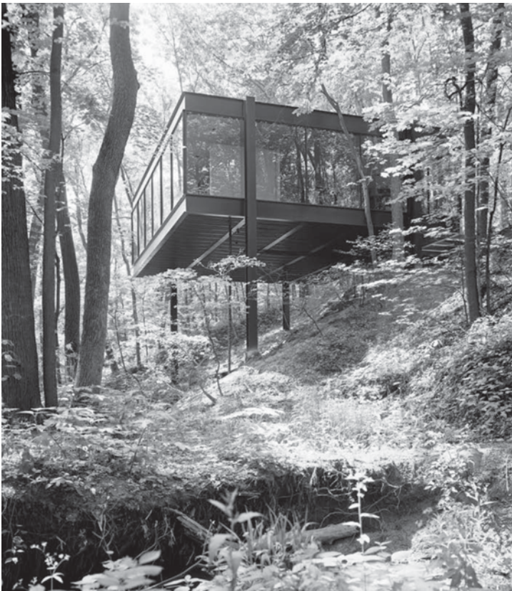
Steel-and-glass Auto Pavilion— built on stilts projecting over ravine 6
