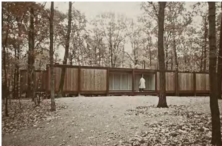
Facade with cypress vertical siding flanking the recessed front entrance 1
