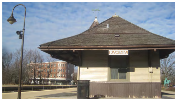
Ravinia Crossing appropriately neighbors the Ravinia Metra Station
