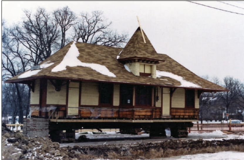
A jacked-up Ravinia Station photograph courtesy Highland Park Archives and Local History Collections.
