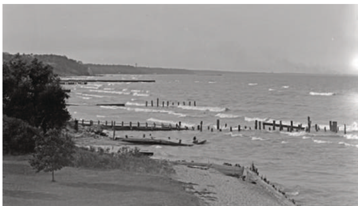
2. Lake Michigan is hard on structures. Ruined piers, circa 1990
